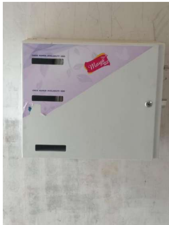
Sanitary pads vending machine and incineration units were installed.
